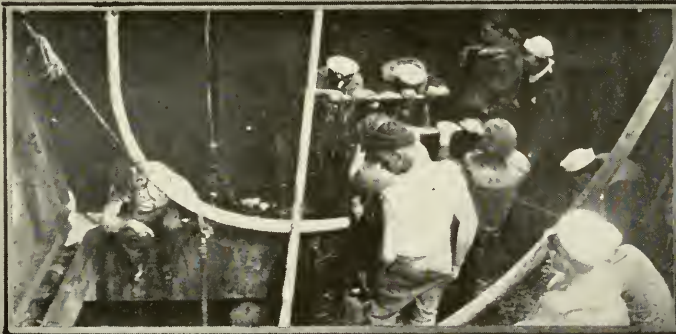
ANOTHER VIEW OF THE PUMPS
